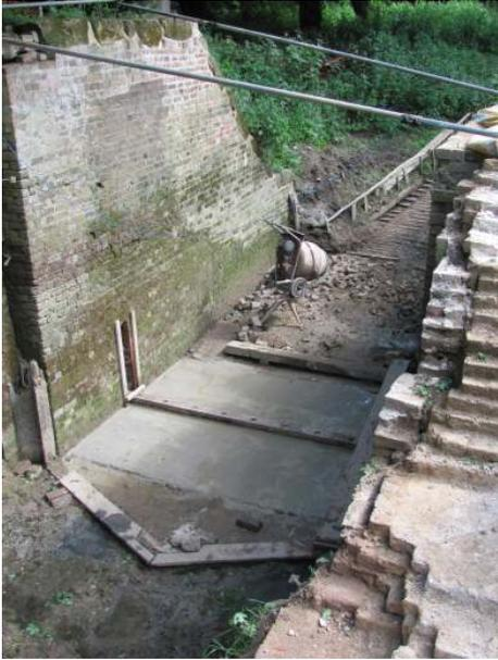
Somehow a day was selected, during some of the most unsettled weather for years. The lock was regularly pumped dry leading up to the chosen day and on Saturday 9<sup>th</sup> June the 'big pour' was completed in a continuous seven hour operation involving most of the regular SORT workforce with some invaluable additional help from three members of the Kent and East Sussex Canal Restoration Group (KESCRG).
