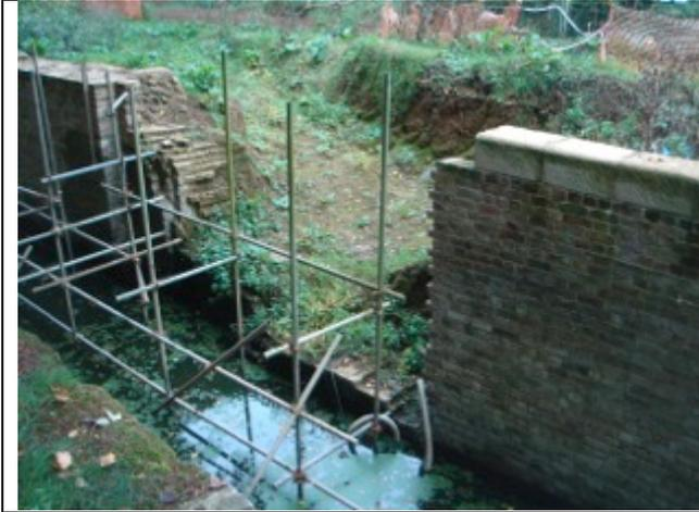
Summer 2014's main task will be to complete the restoration of the west chamber wall at Isfield Lock. Both ends have been done and now we'll do the central section. Preparation for this work will be made over the coming autumn and winter. We'll need to dig out more of the dirt behind the wall – down to invert level, so another six or seven feet or so. Could be dirty work!
