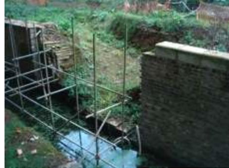
If we just used concrete behind the new area of wall, we might need as much as 50m<sup>3</sup> of concrete. However, we do have lots of broken bricks we can use to reduce the quantity of the concrete, without losing any strength, and save a pile of cash. I expect we will also be finishing off the remaining ground paddle (see below) and the stop plank channels.
