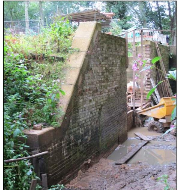
(above) The 5m section of the chamber wall under restoration and (right) the completed west bottom end of the lock with the hole in the background.
