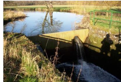
Fletching Mill – steel plate installed at site of collapsed sluice gates to maintain upstream water levels
