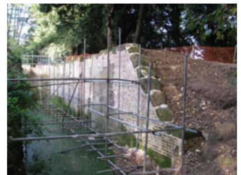
Some of the work already done at Isfield Lock.
